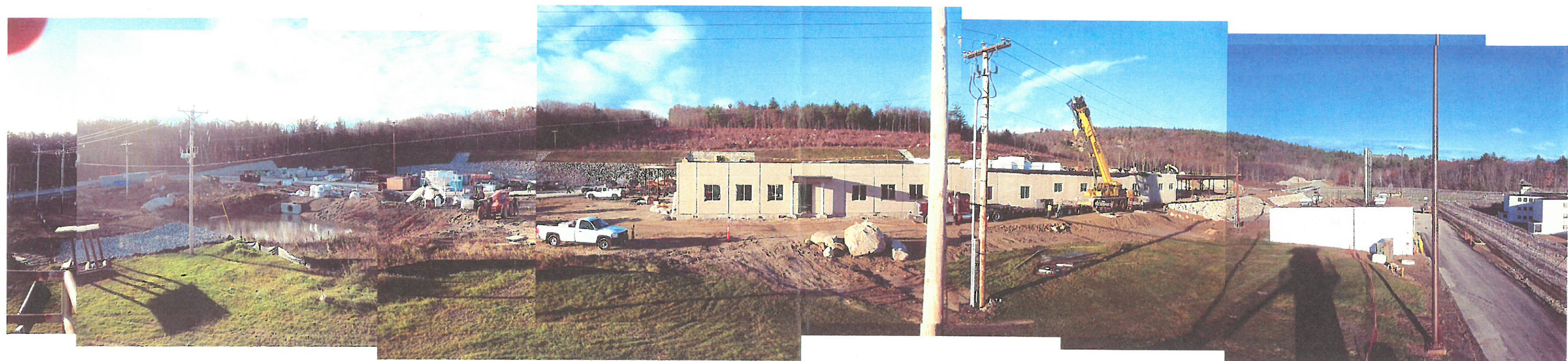
SITE FROM TOWER 1 – 11/17/2016 (GMP2 – Gilbane/Cairns/IES/M-P/J&J/Szetela/Capone/Tightline/Stresscon/Progressive)
