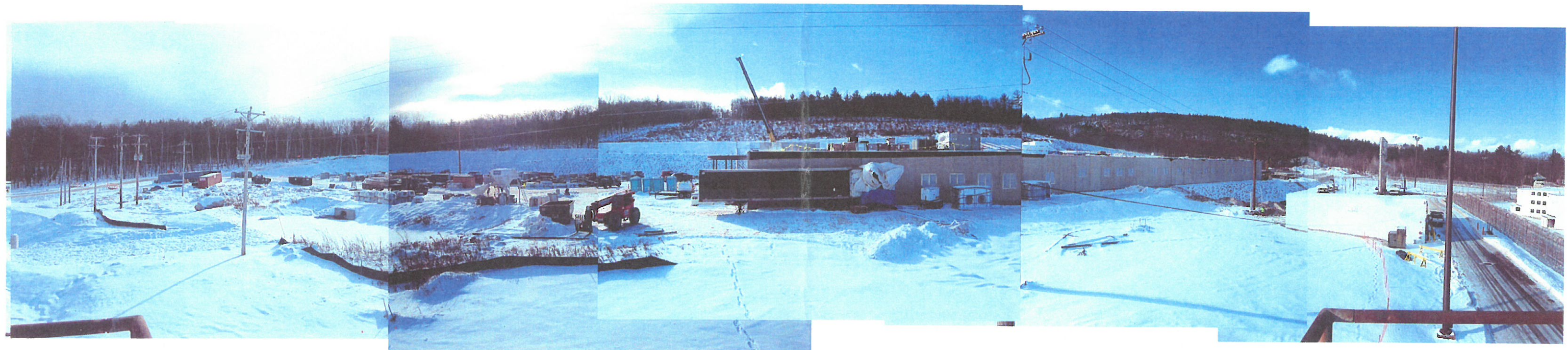
SITE FROM TOWER 1 – 12/15/2016 (GMP2 – Gilbane/Cairns/IES/M-P/J&J/Szetela/Capone/Tightline/Stresscon/Progressive)
