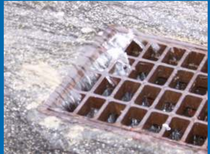
Commercial parking lot runoff, Concord, NH
