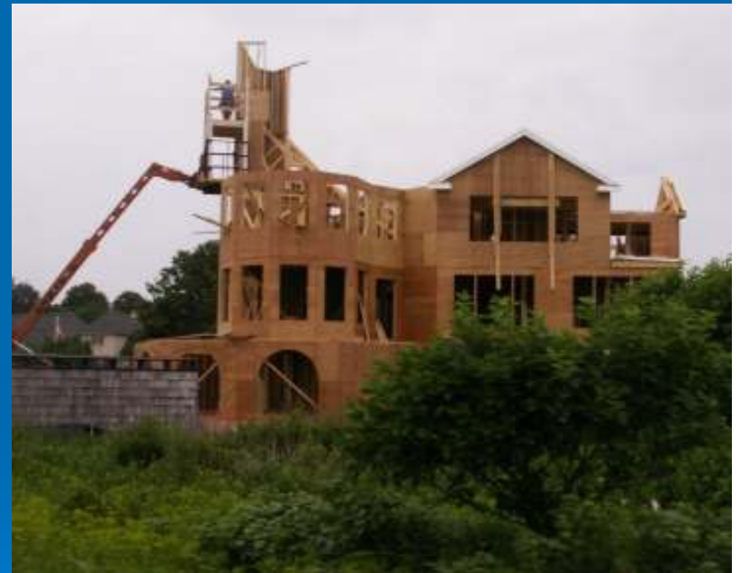
Residential construction, NH Seacoast
