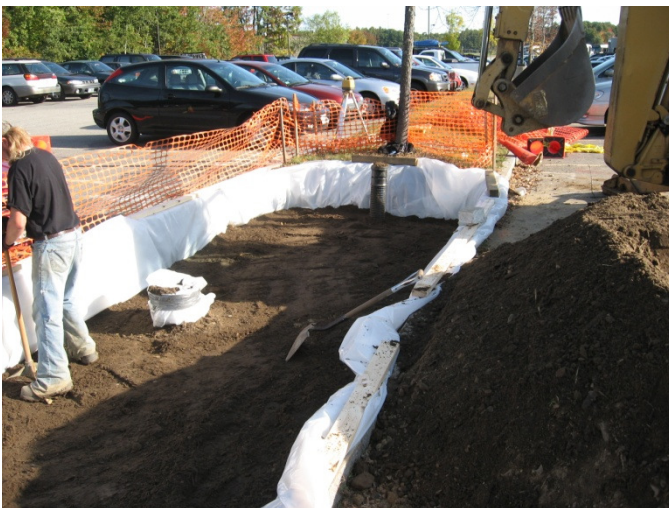
Figure 2: Bioretention retrofit installation at the University of New Hampshire, October, 2008
