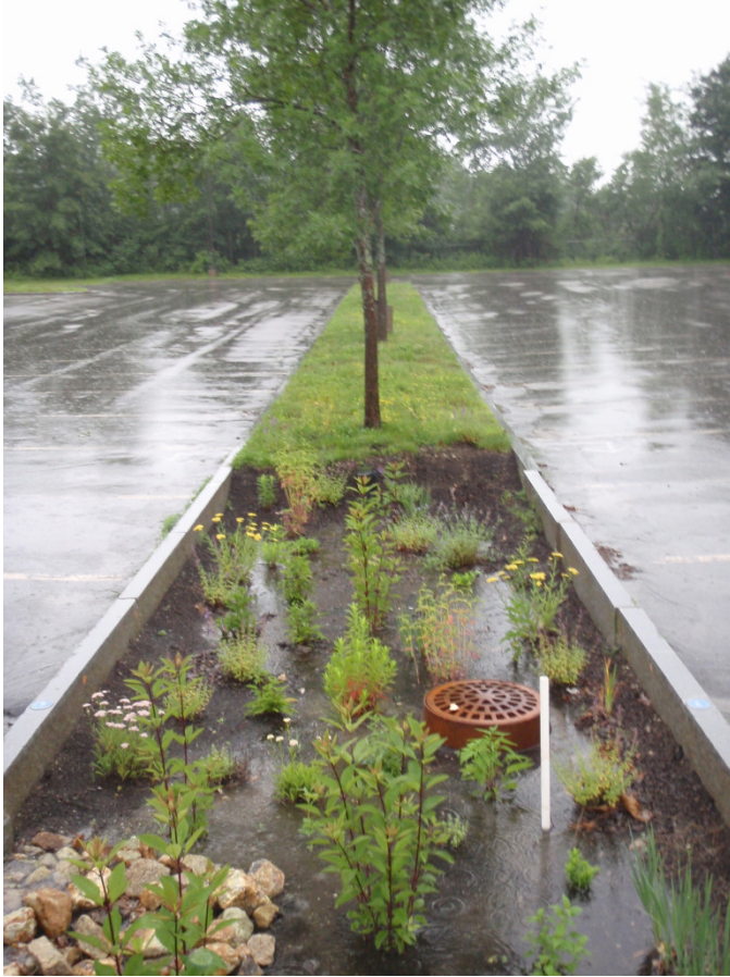
Figure 3: Completed Bioretention Retrofit Installation 2008
