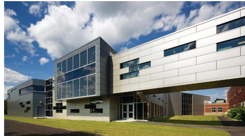
MCC external including replacement of old windows for greater energy efficiency
