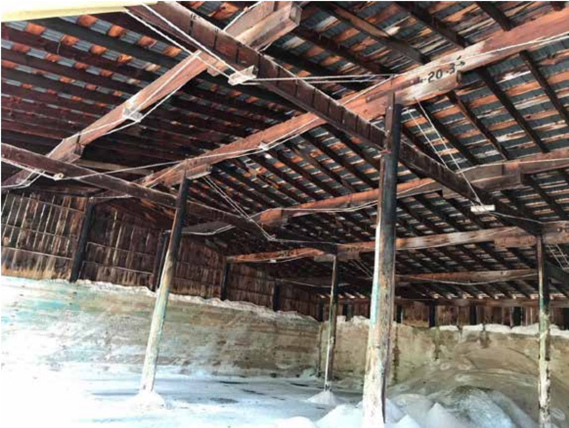
Photo 5: Lincoln (115) – Salt Shed internal structure
