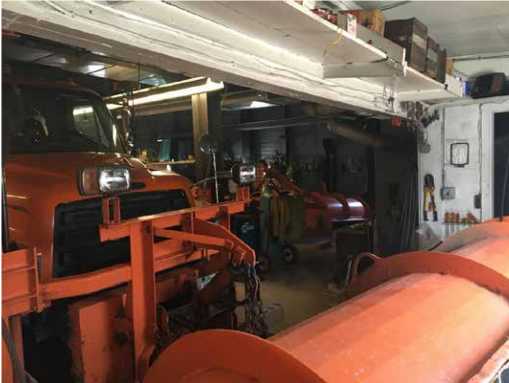
Photo-5: View of inadequate headspace over parked vehicle.
