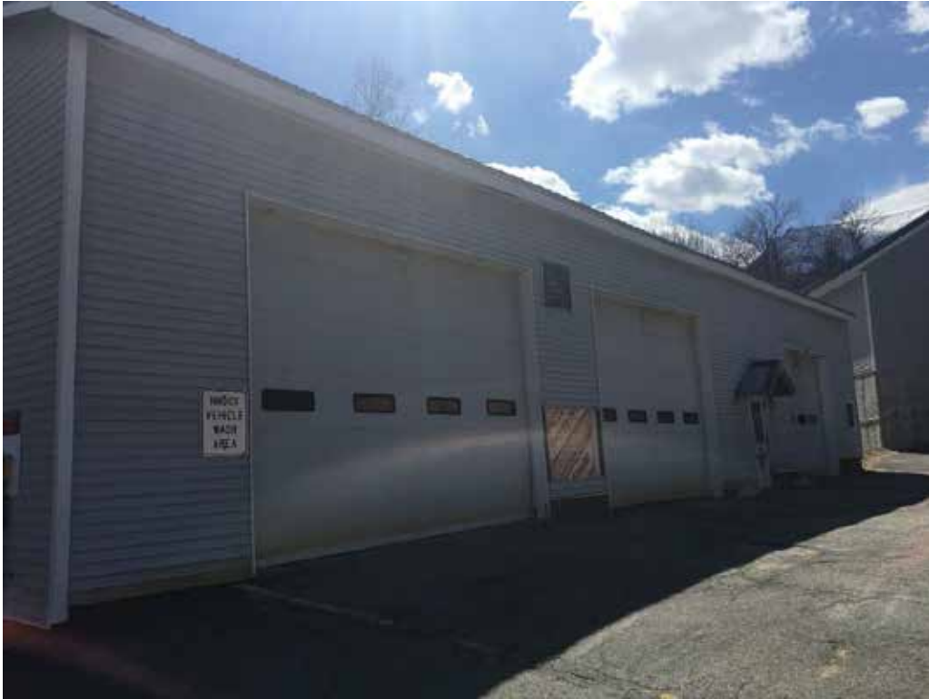
Photo-1: Front view of existing patrol shed. Garage doors are in need of replacement and are undersized to safely accommodate the vehicles and equipment.
