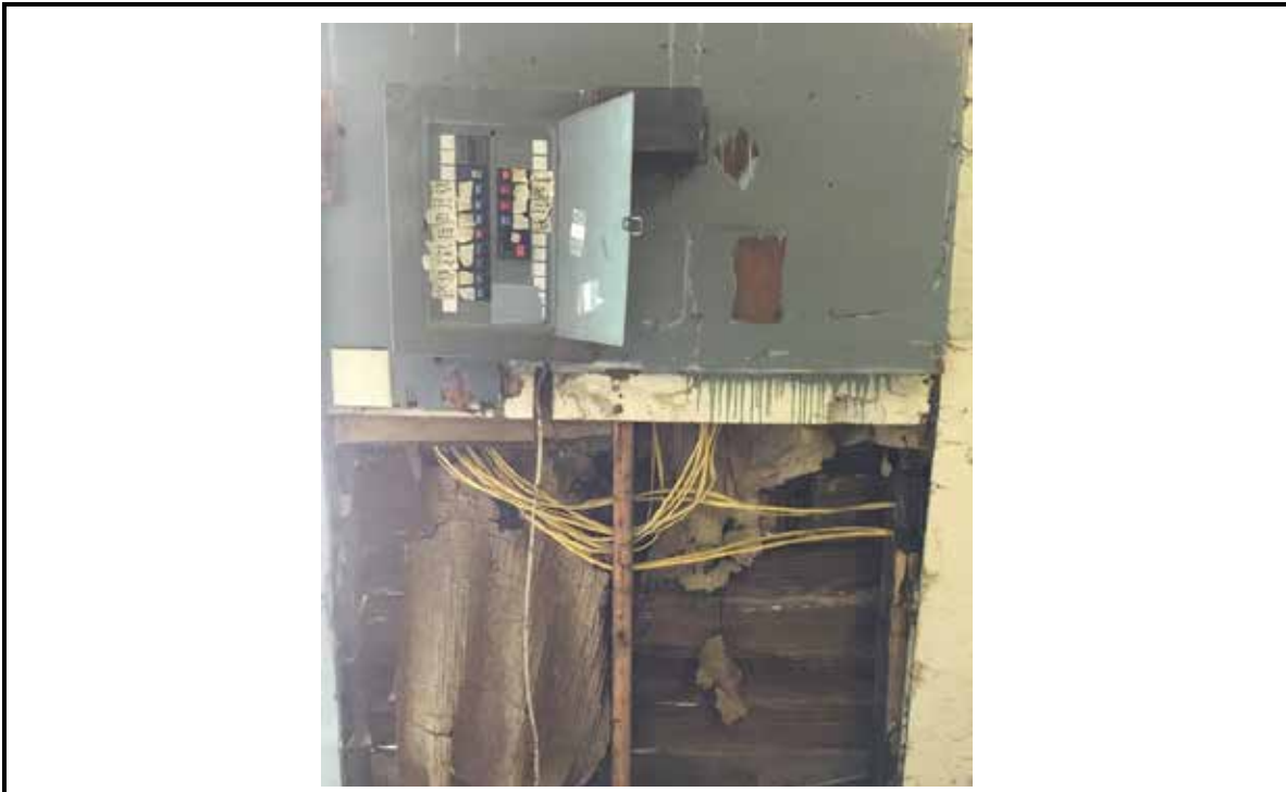
Figure 4: Inside of Sidewall
