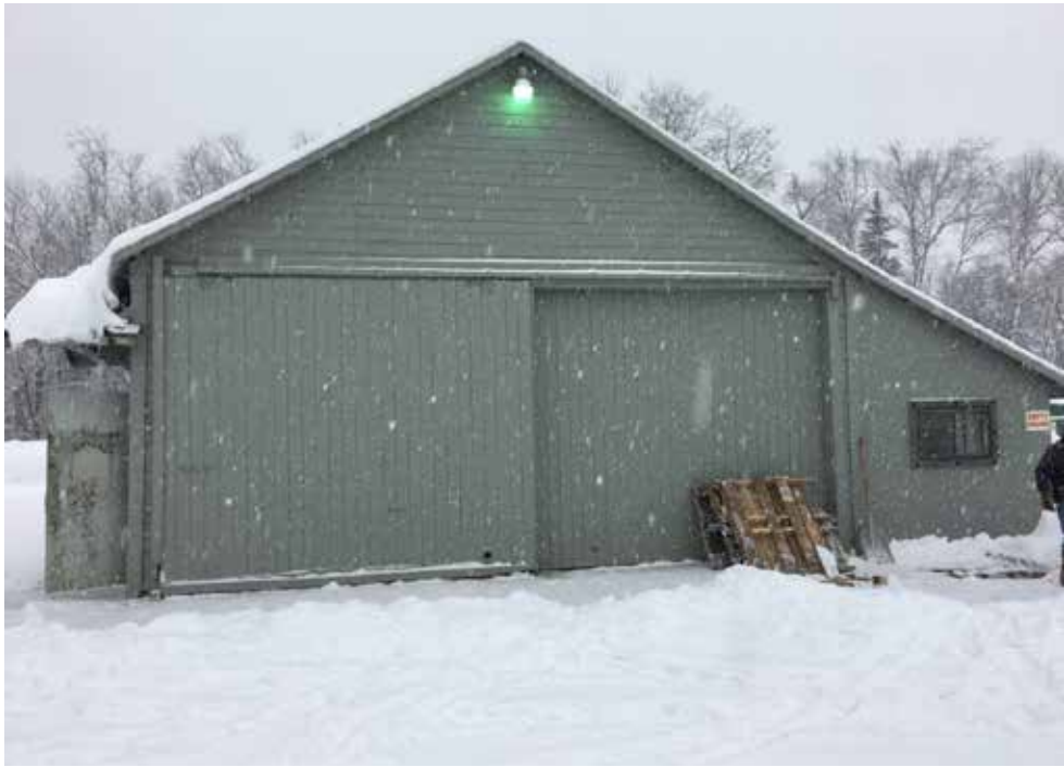
Figure 1: Front View of Building
