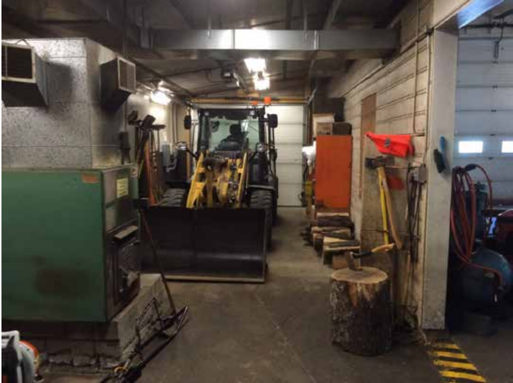
PS512 Londonderry Interior View of Tractor Bay with wood burning furnace
