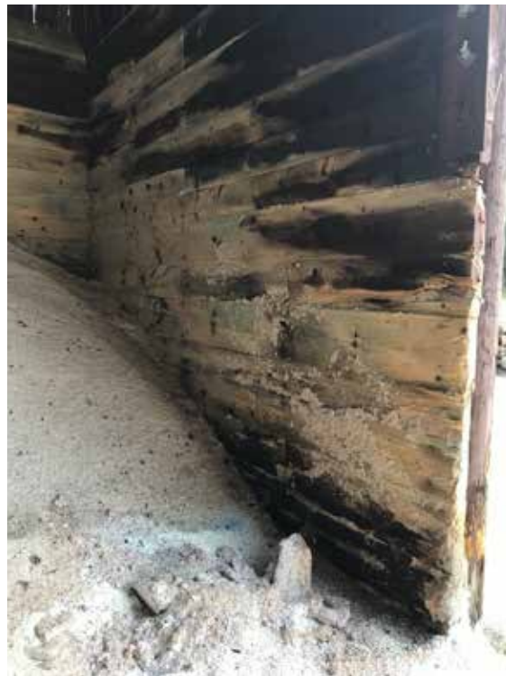
Photo 9: Belmont (314)- Deteriorated wall condition
