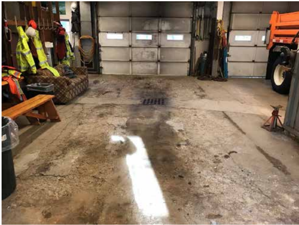
PS510 Milford Interior View of Loader Bay with low clearance
