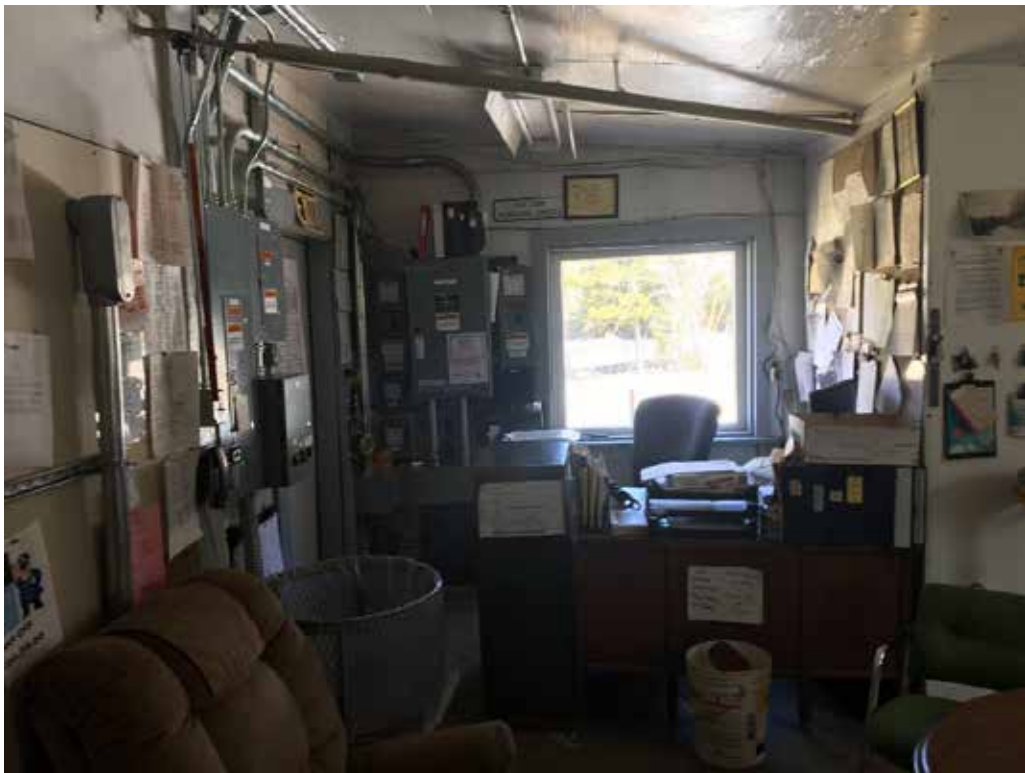
Photo-12: View of crew quarters / Office space and electrical breaker room.
