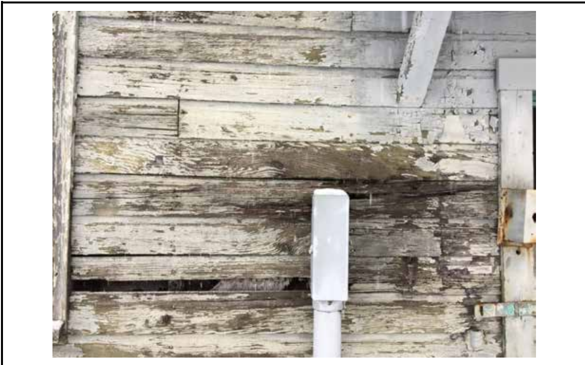
Figure 3: Close up of Sidewall (Exterior)
