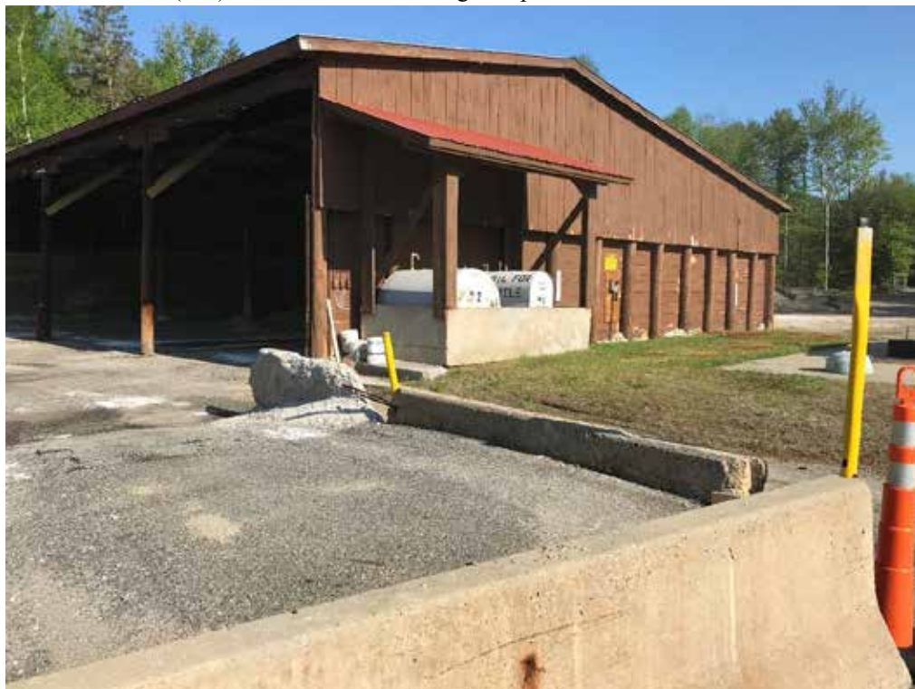
Photo 4: Lincoln (115) – Salt Shed and Loading Ramp
