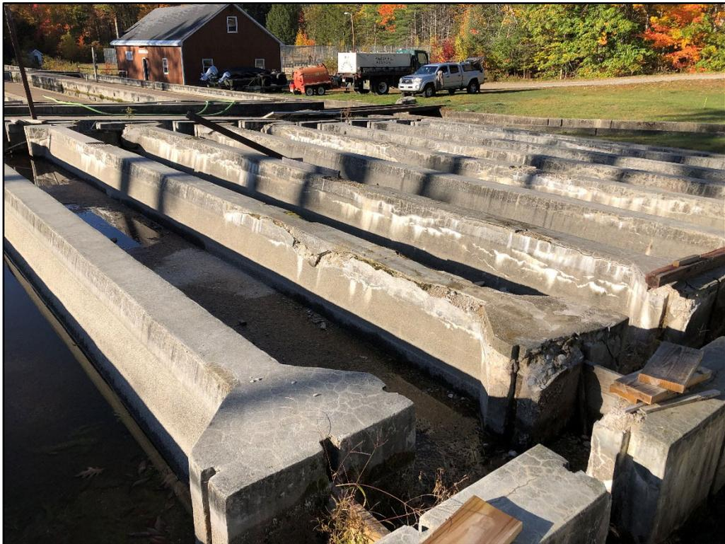
*Figure 2 - Raceway A Concrete Damages*
