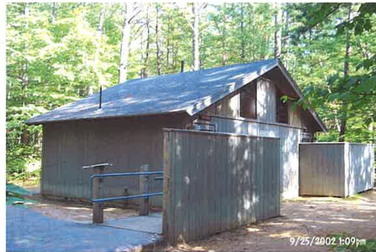
White Lake Toilet Building #2 (WHT11)
