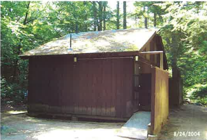
Pawtuckaway Toilet Building #2 (PAW10)
