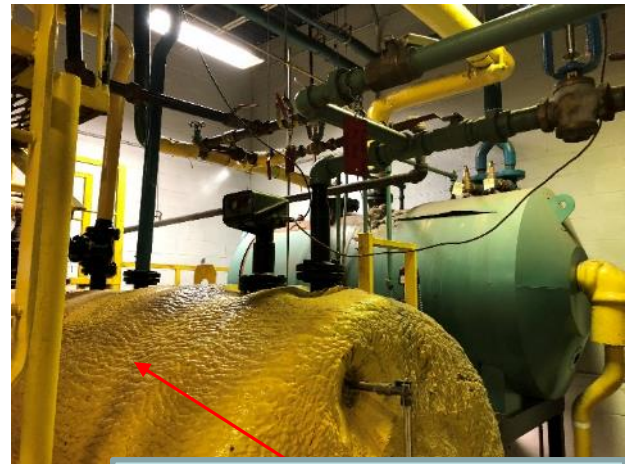
Temporary Insulation
