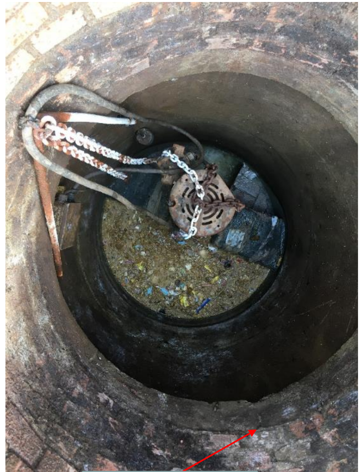
Old brick work
