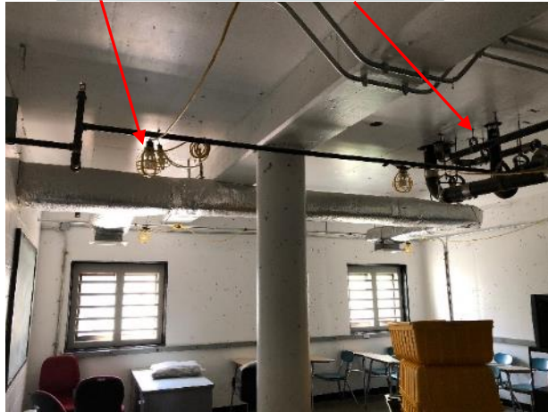
Temporary wiring
