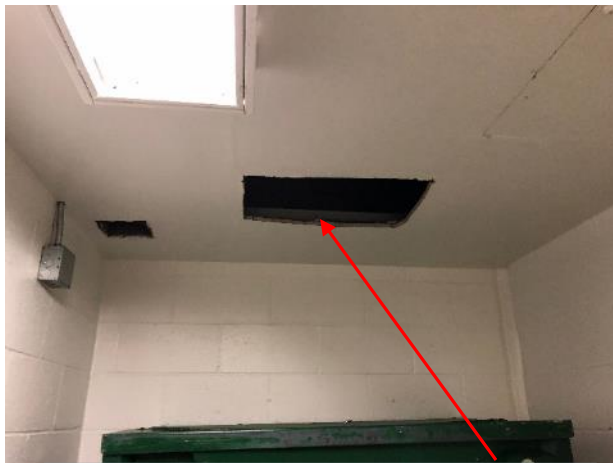
Holes cut to release water
