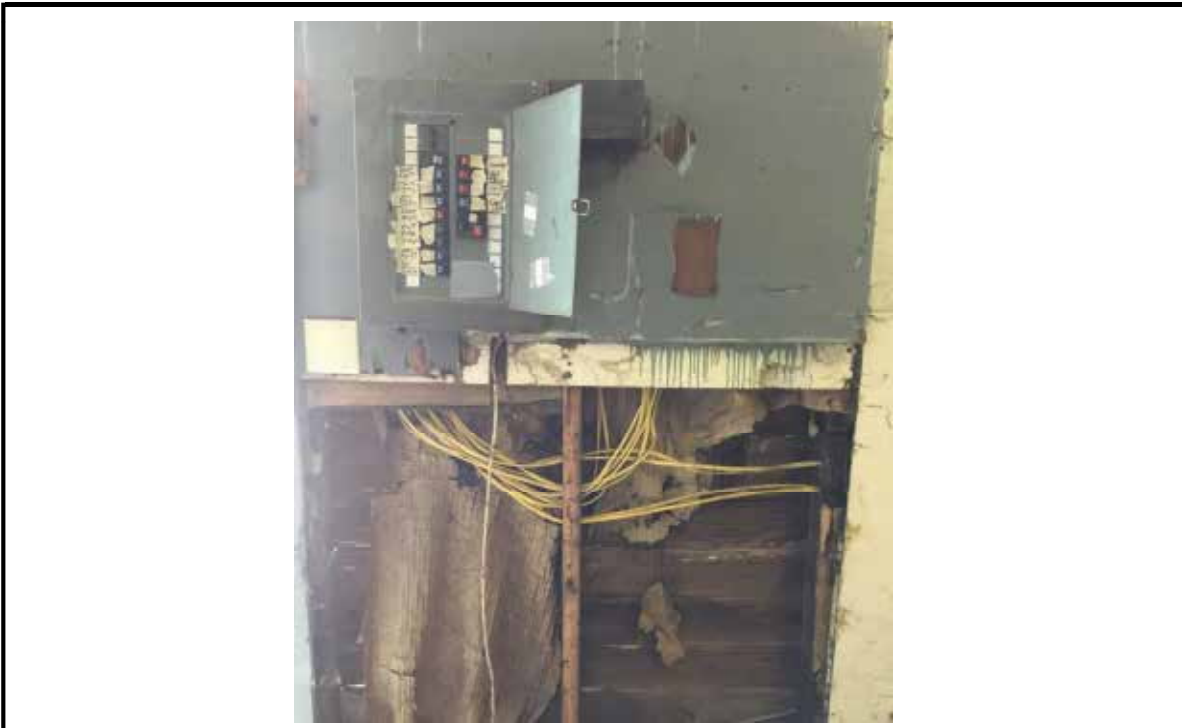
Figure 4: Inside of Sidewall
