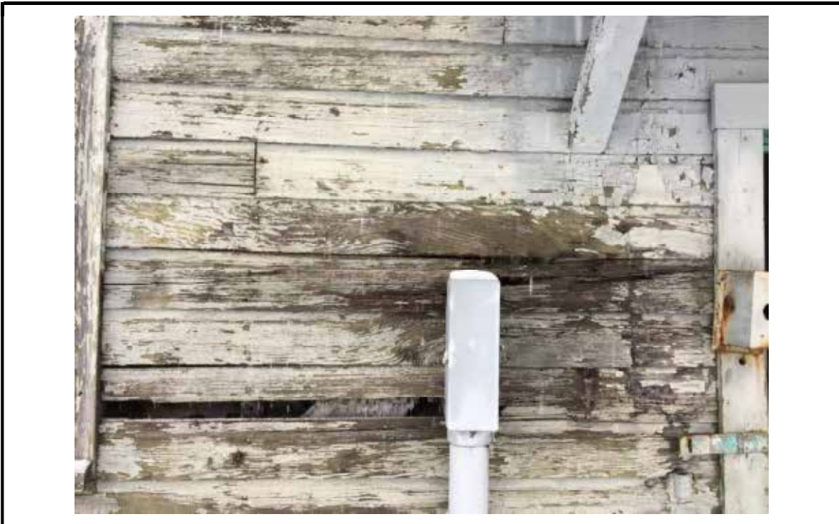
Figure 3: Close up of Sidewall (Exterior)
