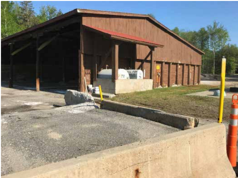
Photo 4: Lincoln (115) – Salt Shed and Loading Ramp
