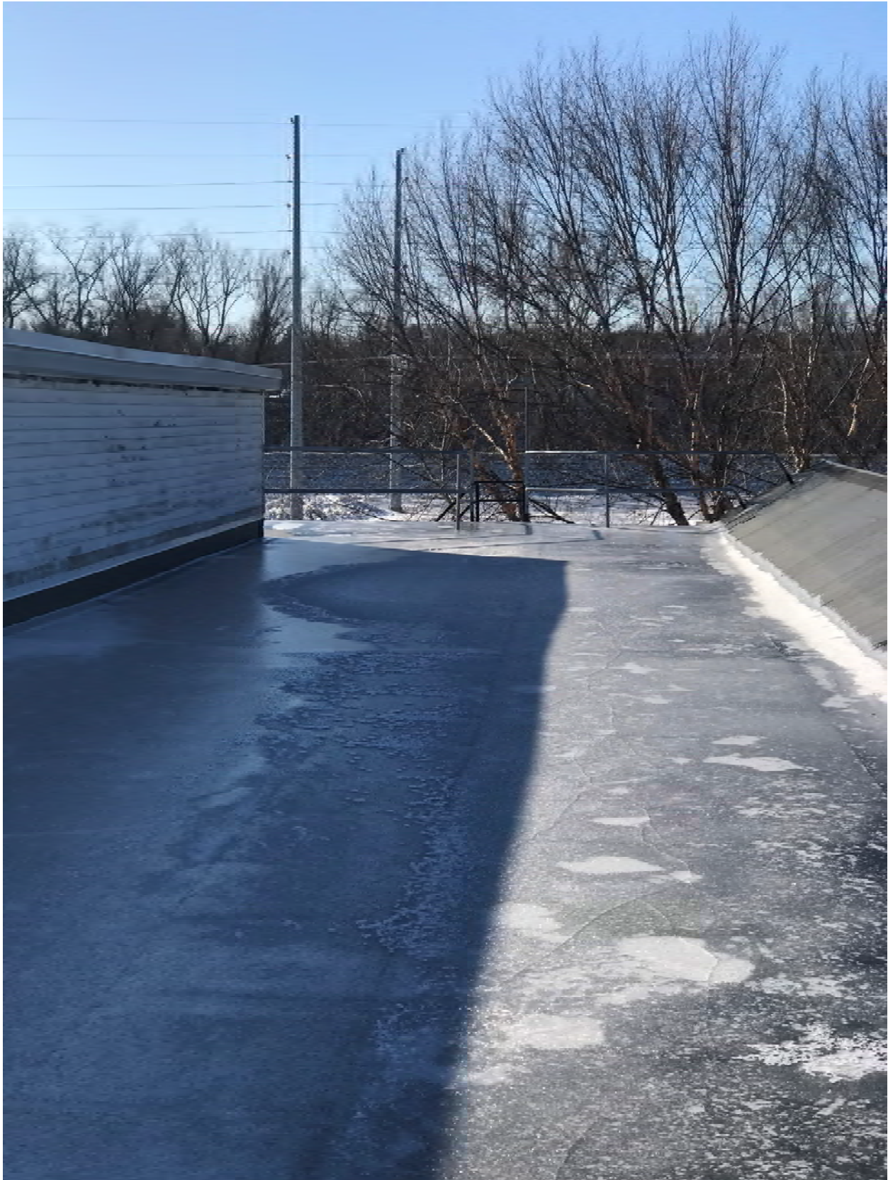
Figure 11 - Path from Doors to Fire Escape
