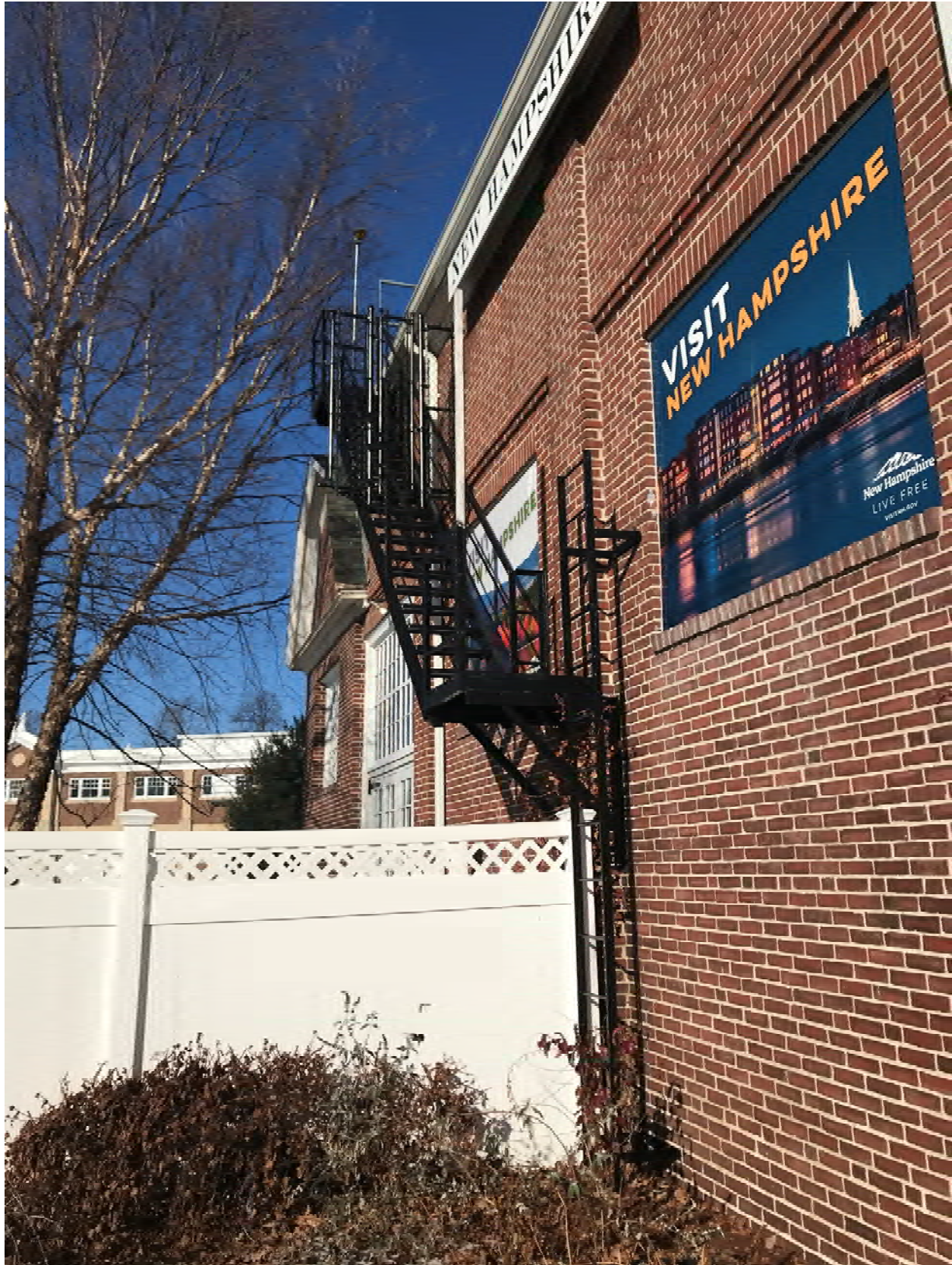
Figure 13 - Fire Escape at Rear of Building
