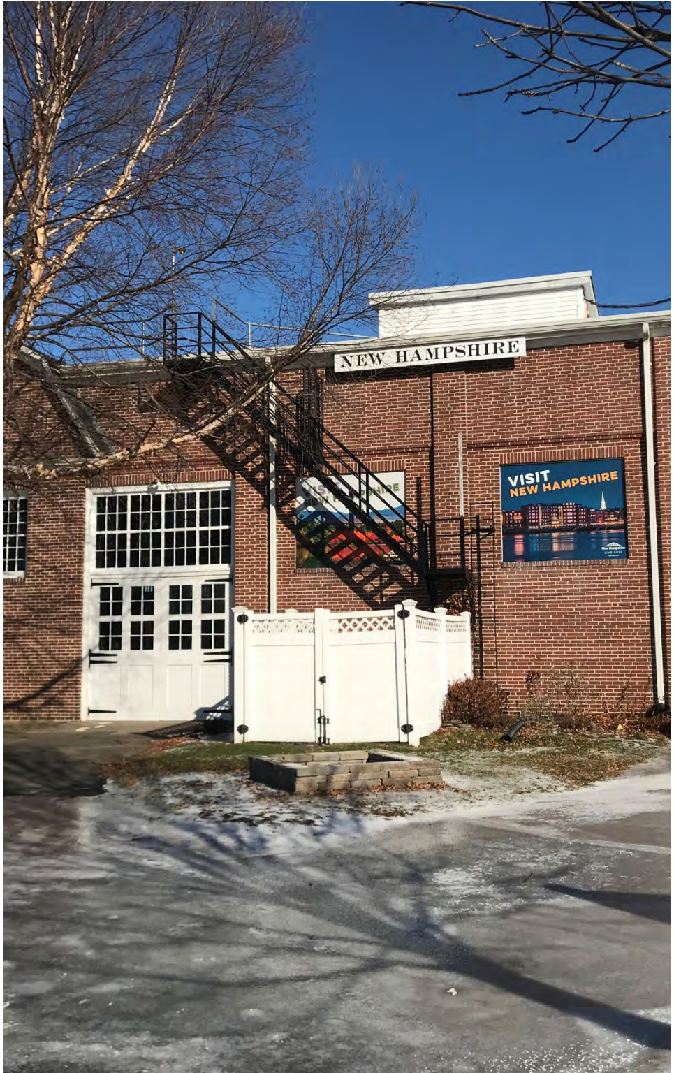
Figure 12 - Fire Escape at Rear of Building
