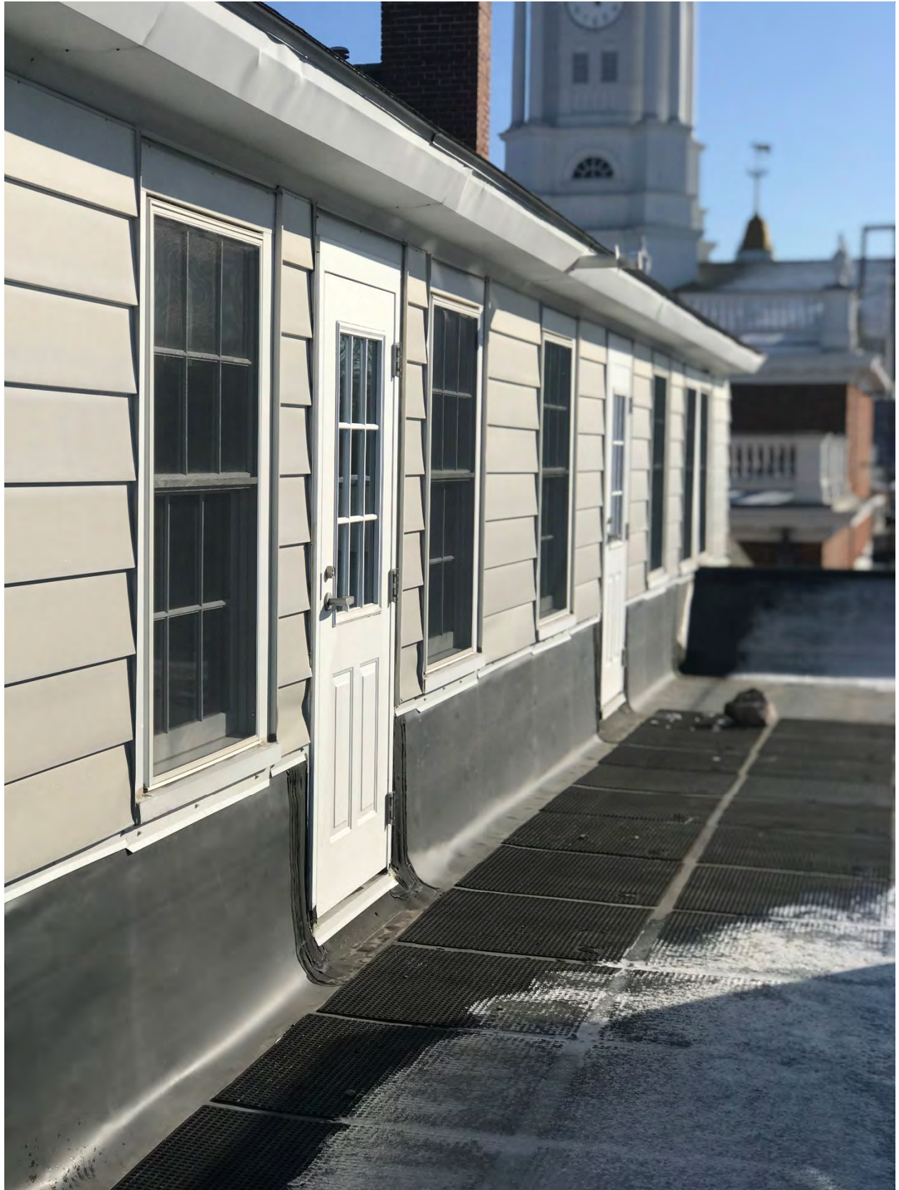
Figure 10 - Exit Doors to Roof (Exterior)
